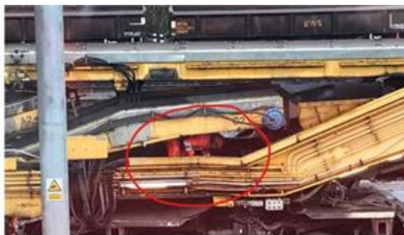
Image shows the operative working inside the BCS system.
